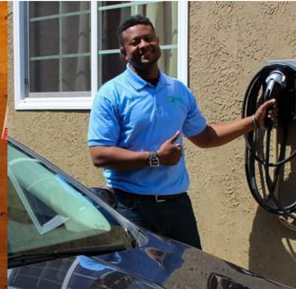
EV Supply Equipment
